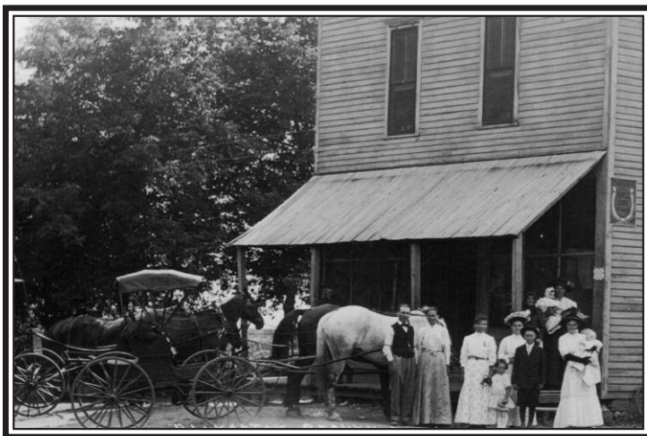
The Kartak General Store located in Bechyn in Henryville Township. (Photo courtesy of Janice Olsen)
