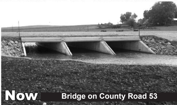
Bridge on County Road 53
