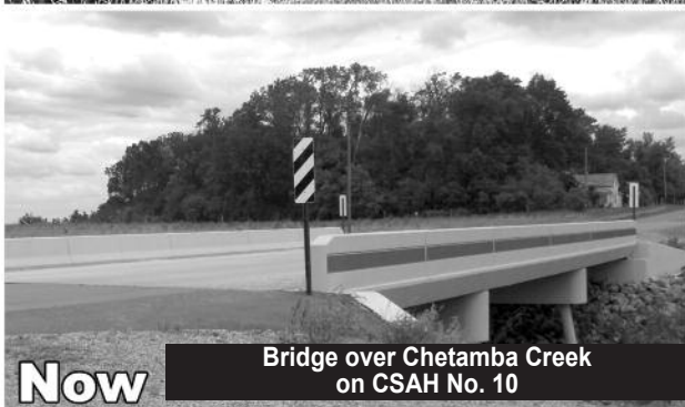
Bridge over Chetamba Creek on CSAH No. 10
